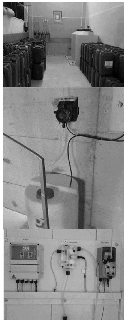
**Figure 3.** Drinking water sodium hypochlorite system
